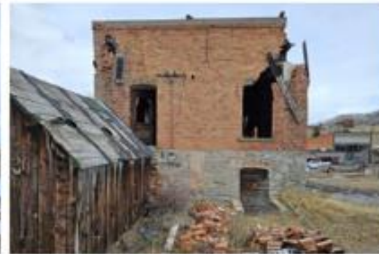
STONEWALL HALL, SOUTH ELEVATION
