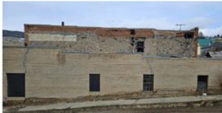
STONEWALL HALL, WEST ELEVATION. DUDLEY IN FOREGROUND
