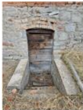
REAR (SOUTH) ENTRY
