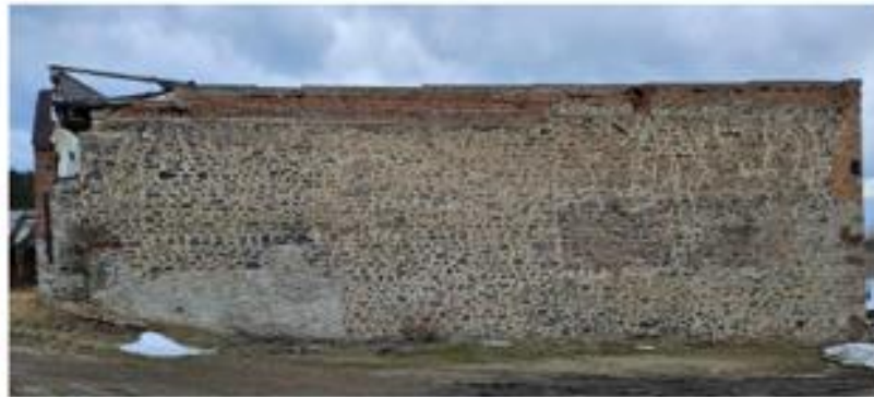
STONEWALL HALL, EAST ELEVATION
