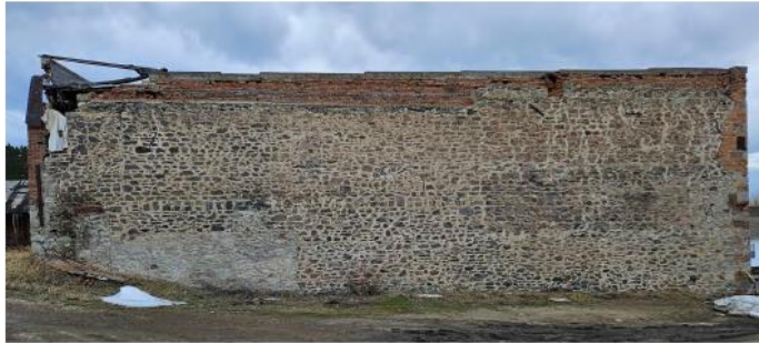
STONEWALL HALL, EAST ELEVATION
