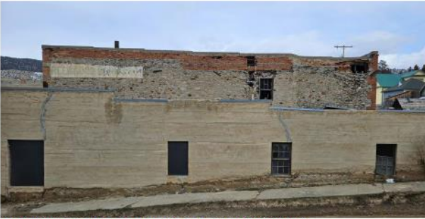
STONEWALL HALL, WEST ELEVATION. DUDLEY IN FOREGROUND
