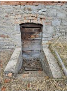
REAR (SOUTH) ENTRY
