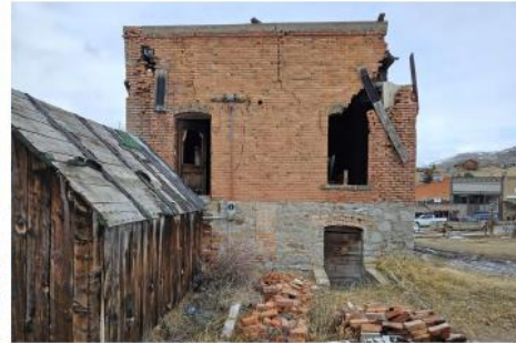
STONEWALL HALL, SOUTH ELEVATION
